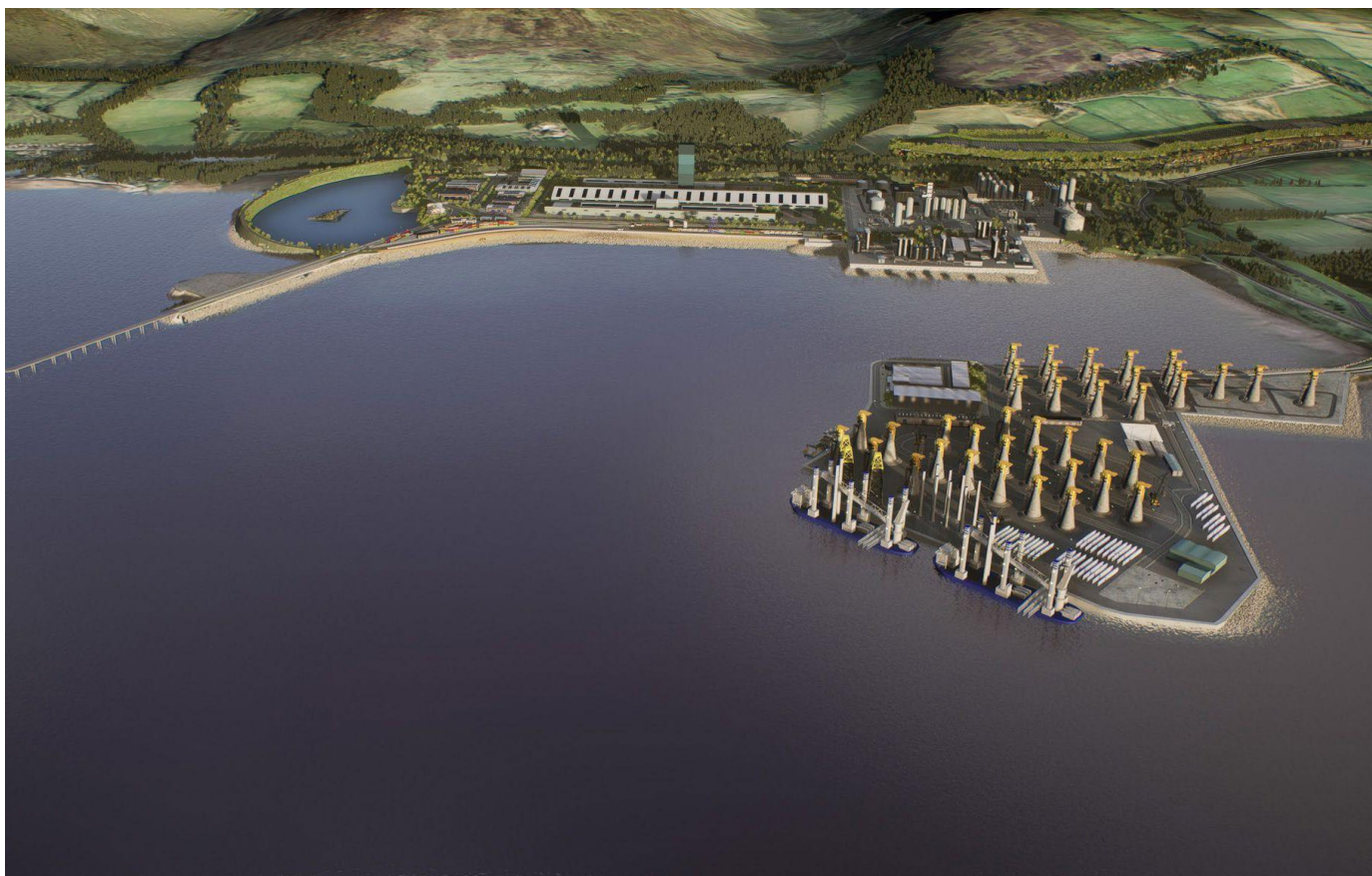
THE DEEP CHANNEL AND MILE-LONG JETTY ALLOWS SHIPS OF ANY SIZE TO DOCK AT THE TERMINAL. IMAGE SOURCE, PEEL PORTS
